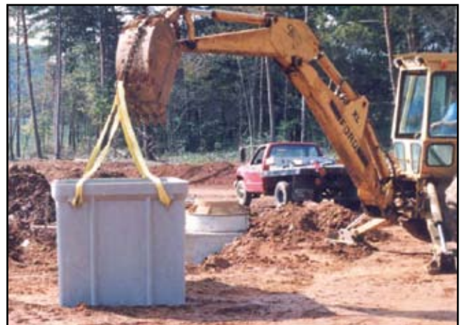
Lift and position enclosure with backhoe (4.03).
